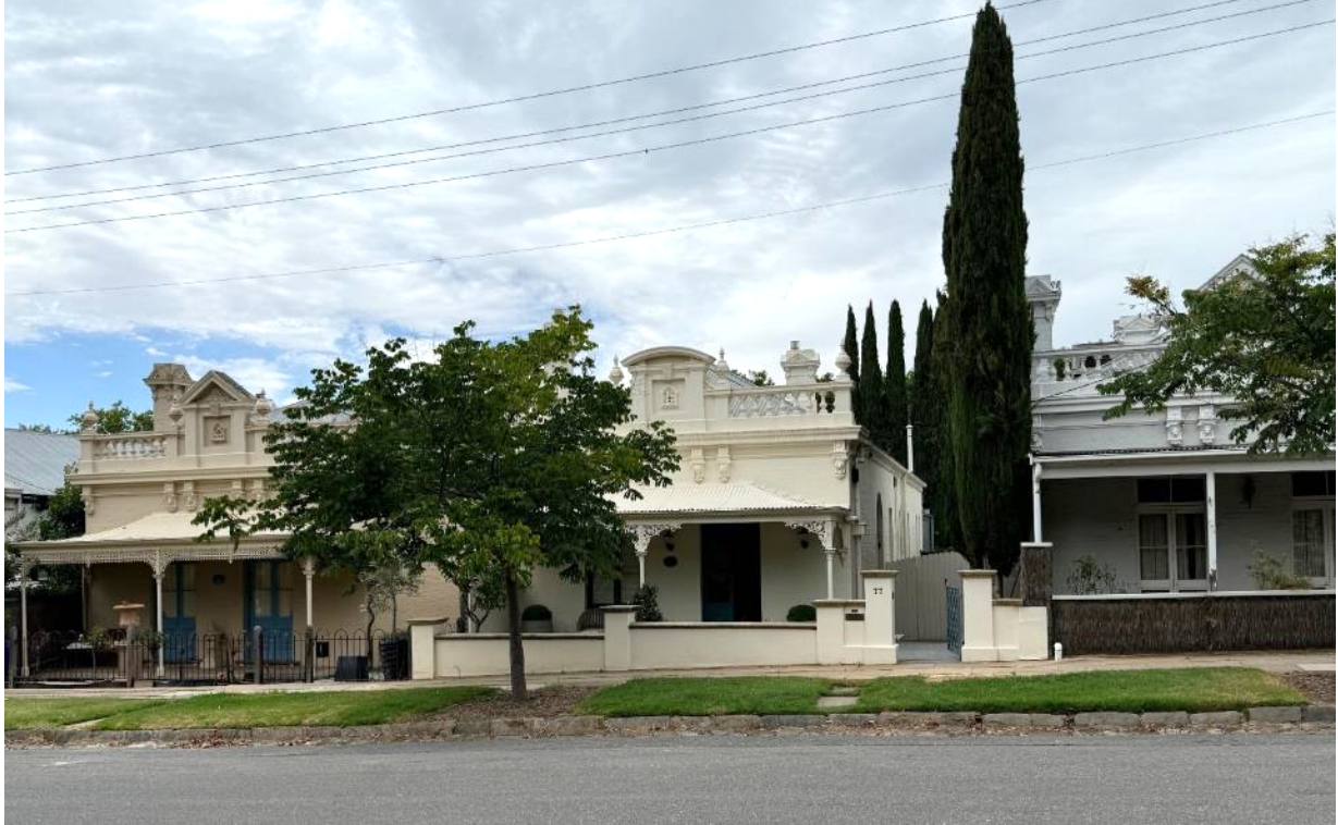
Photo 3.1 – View of the subject site
